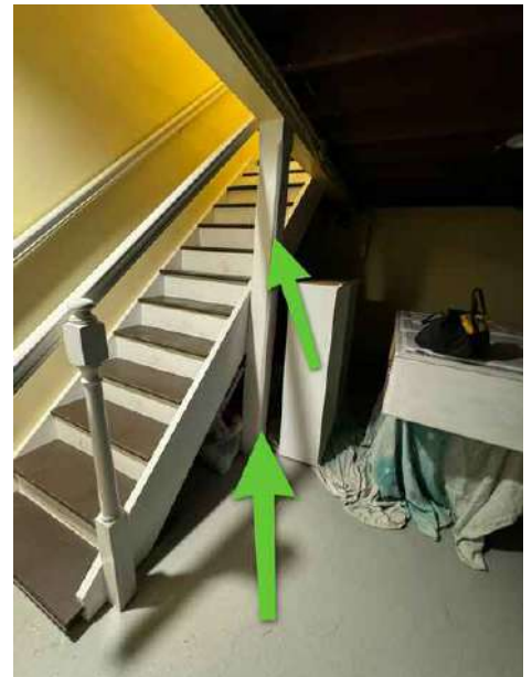
Support column in basement
